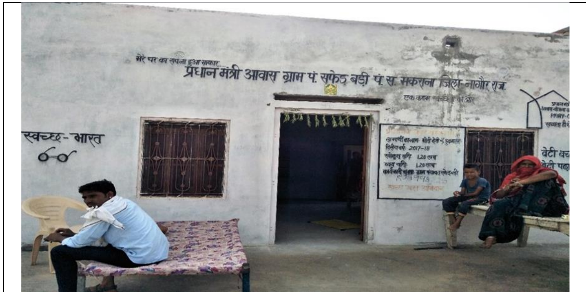
RCC roofing in Rajasthan
