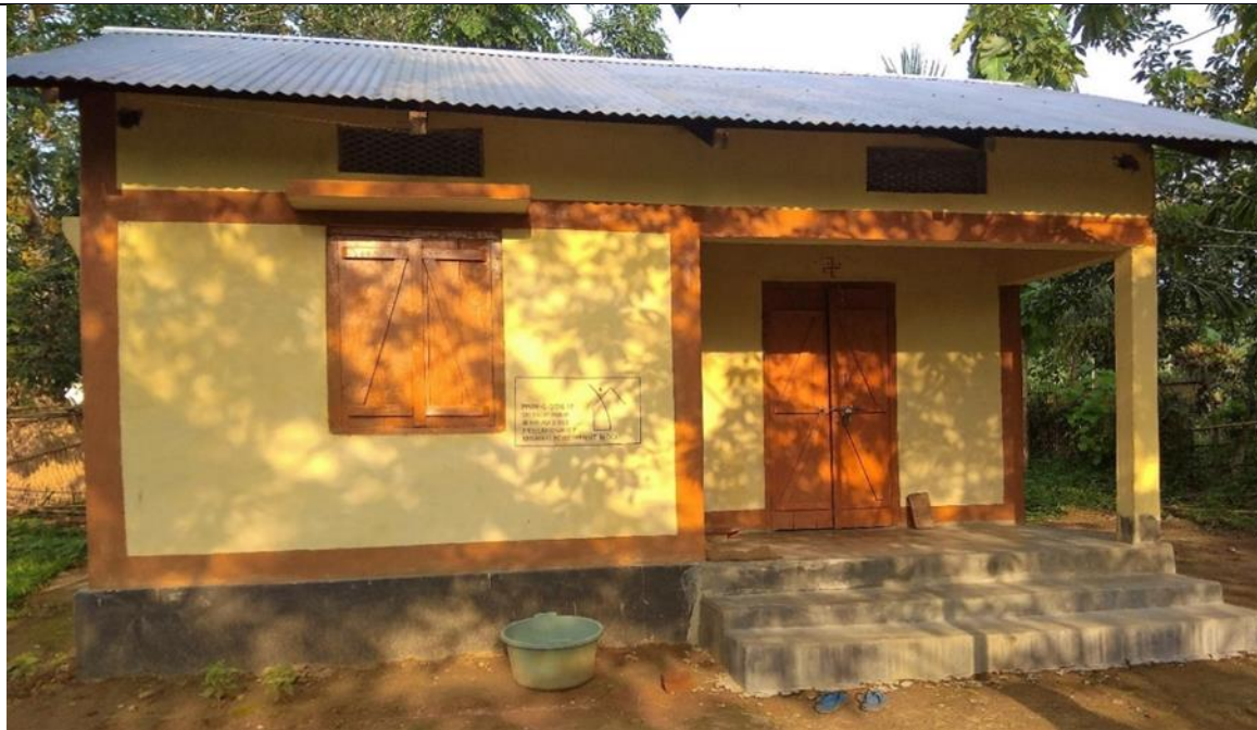
CGI sheet roofing in Assam
