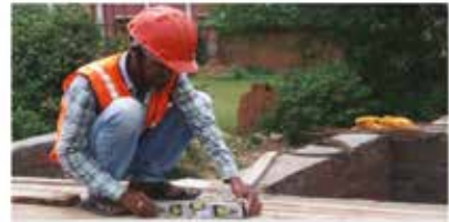
Leveling of Shuttering
