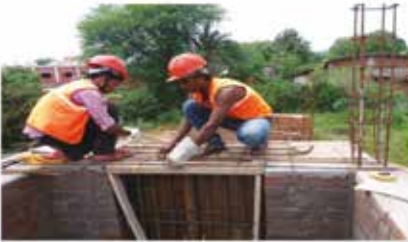
Placing of reinforcement steel
